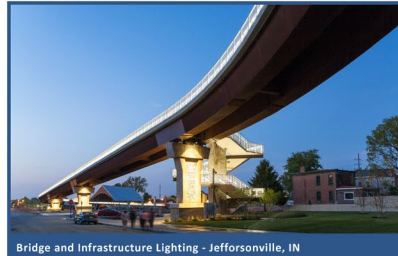
Bridge and Infrastructure Lighting - Jeffersonville, IN
