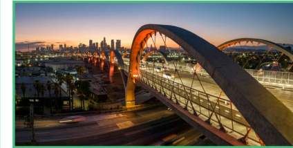
Sixth Street Viaduct Replacement – Los Angeles, CA
