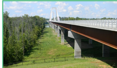
East End Bridge – Louisville, KY
