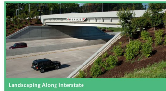
Landscaping Along Interstate
