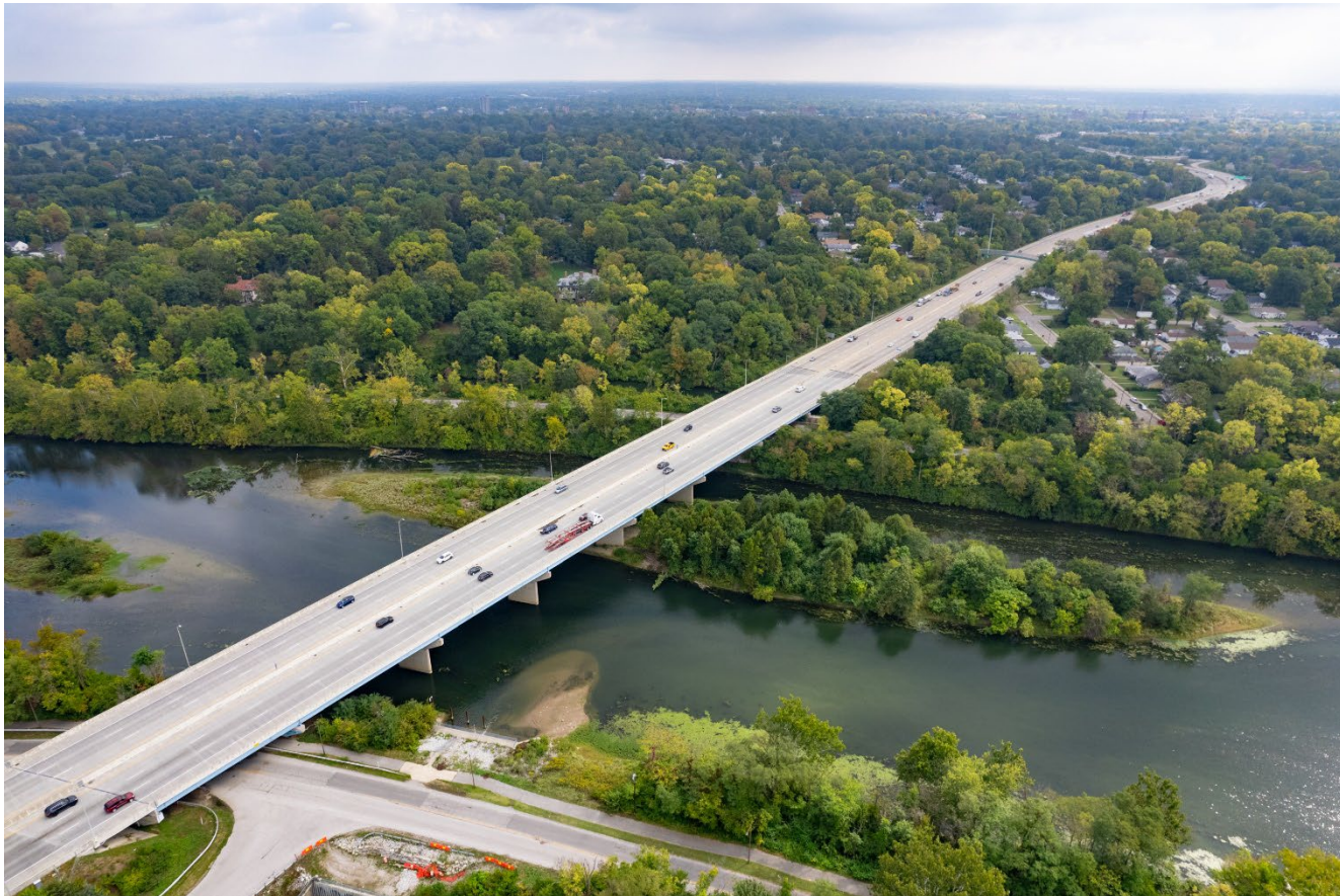
Figure 26. I-65 over the White River
