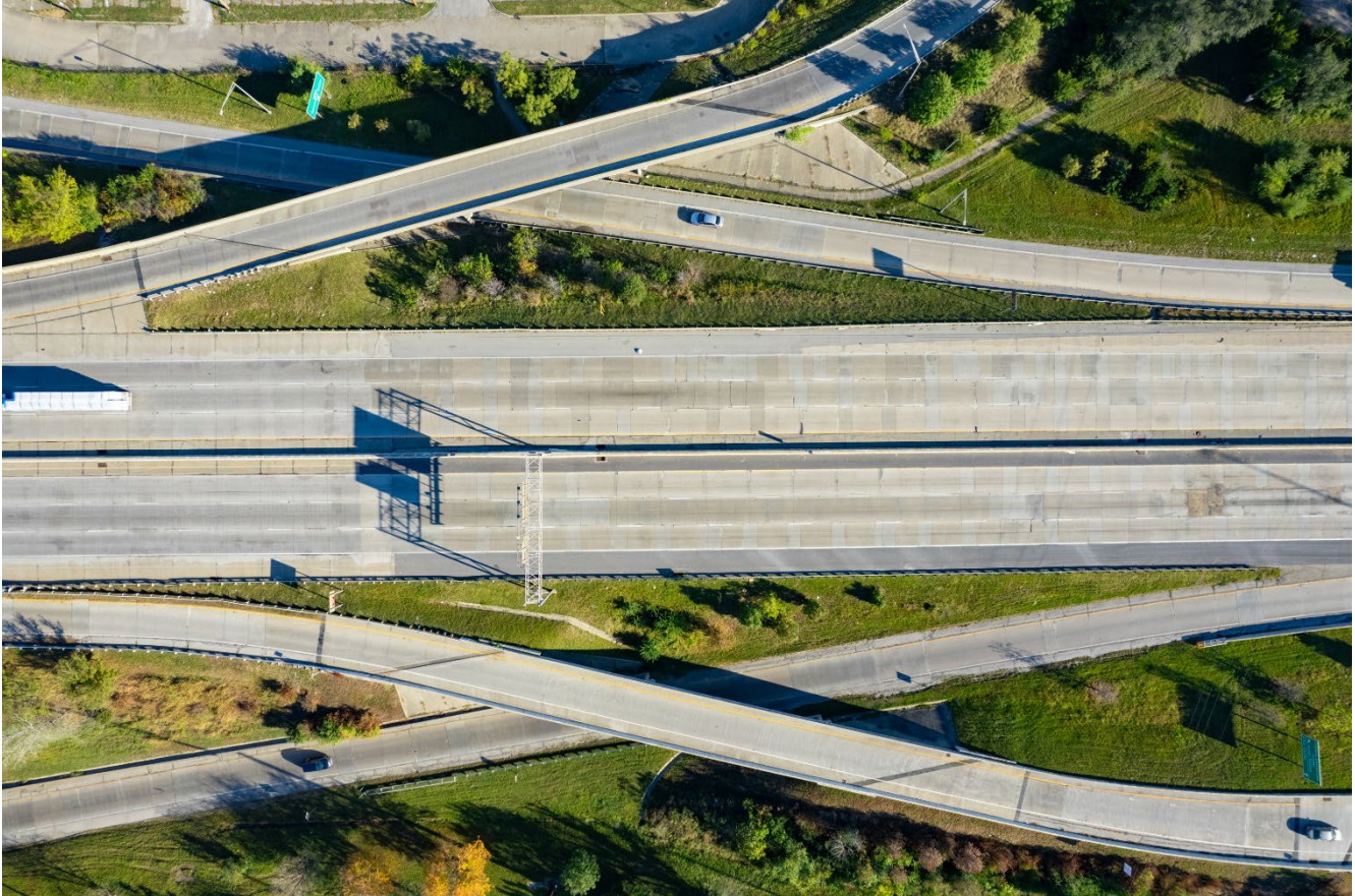
Figure 2. I-70 and Access Ramps East of South Missouri Street
