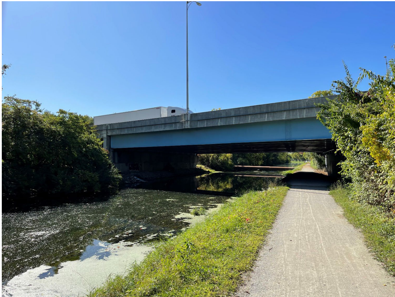
Figure 27. I-65 over the Central Canal and the Canal Towpath
