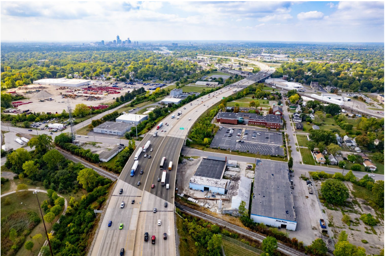
Figure 13. 70 E Spoke at the North Sherman Drive Crossing
