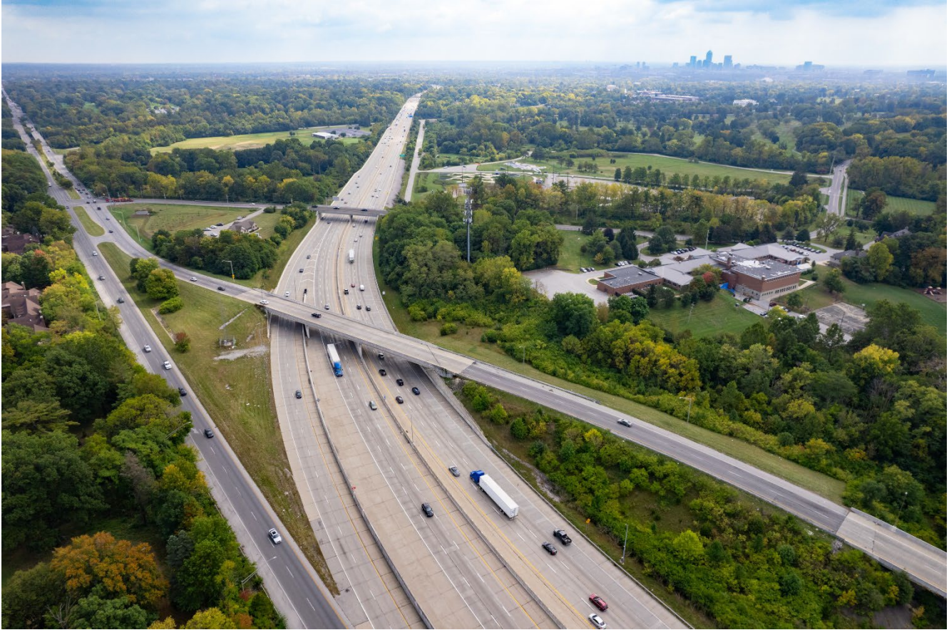
Figure 11. I-65 at 38 th Street and Cold Spring School
