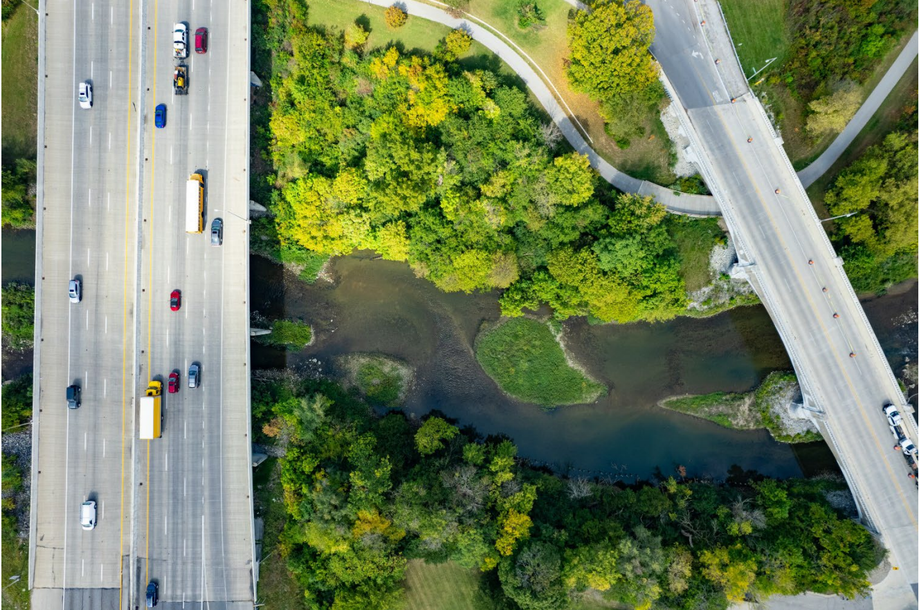
Figure 25. I-65 over Fall Creek
