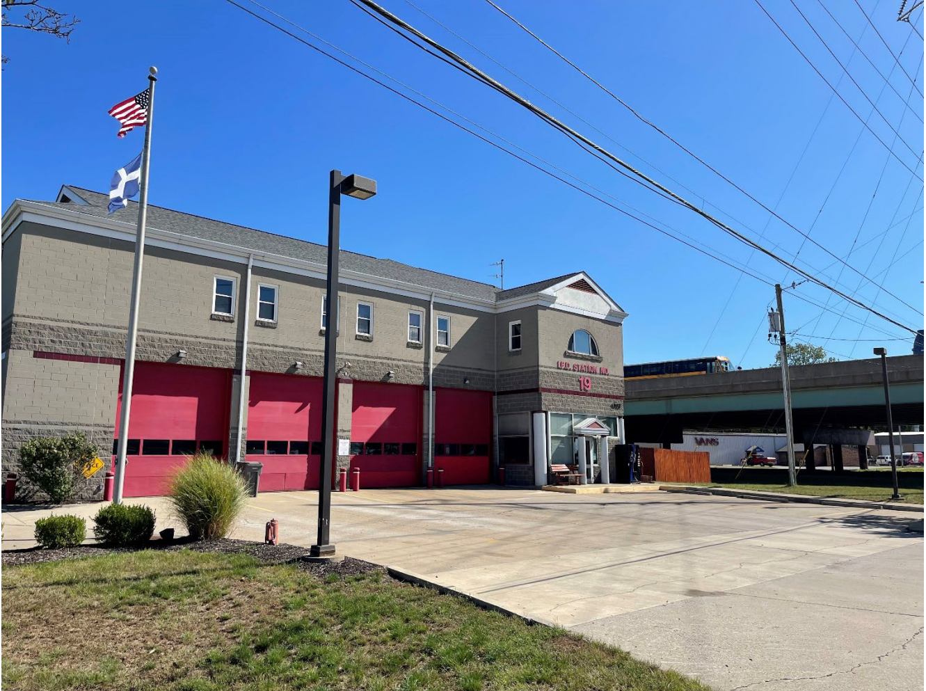
Figure 21. Indianapolis Fire Department Station No. 19
