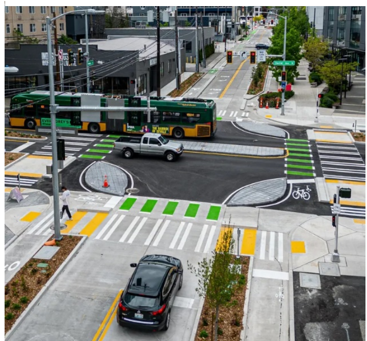
Figure 15: Example of a Local Road Intersection Improvement in Seattle, WA
